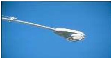
**Example of a fully cutoff Streetlight fixture**
